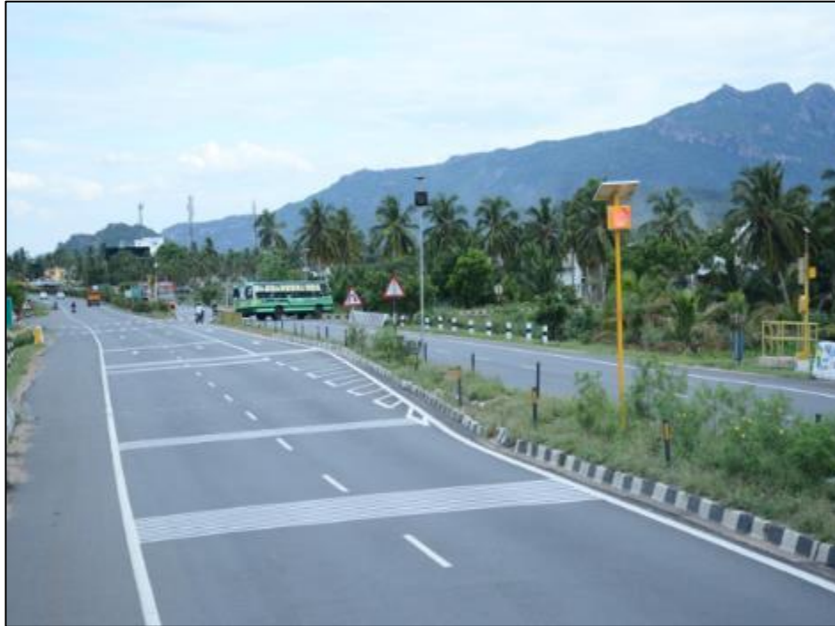
Figure 8-1 : General Project Condition
