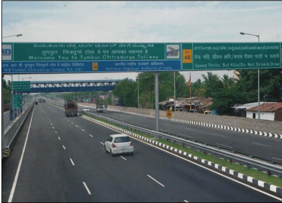
Figure 8-1 : General Condition of project road
