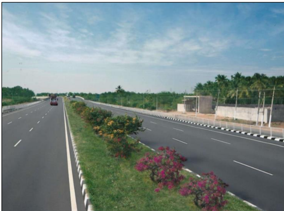
Figure 8-2 : General Condition of project road.
