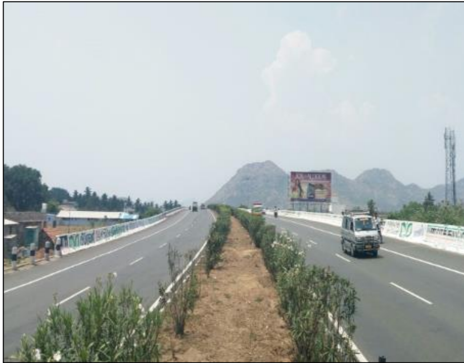
Figure 8-3 General Project Condition
